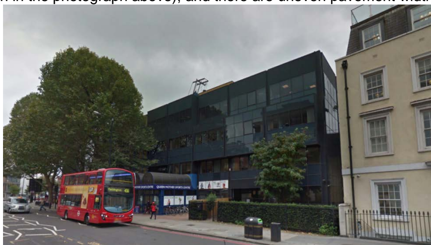
Figure 2.3 Sports Centre frontage and offices, Vauxhall Bridge Road 3
