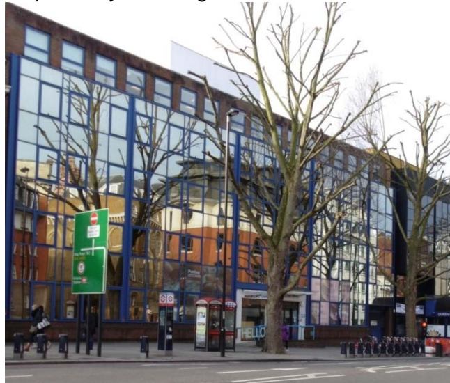
Figure 5.10 No.215 Vauxhall Bridge Road
